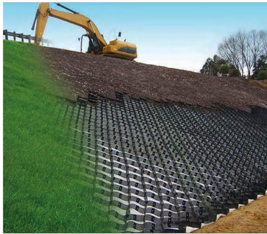
Erosion control webbing for batters greater than 1:3
